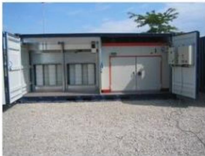
✔ 2. exterieur cabine mobile
